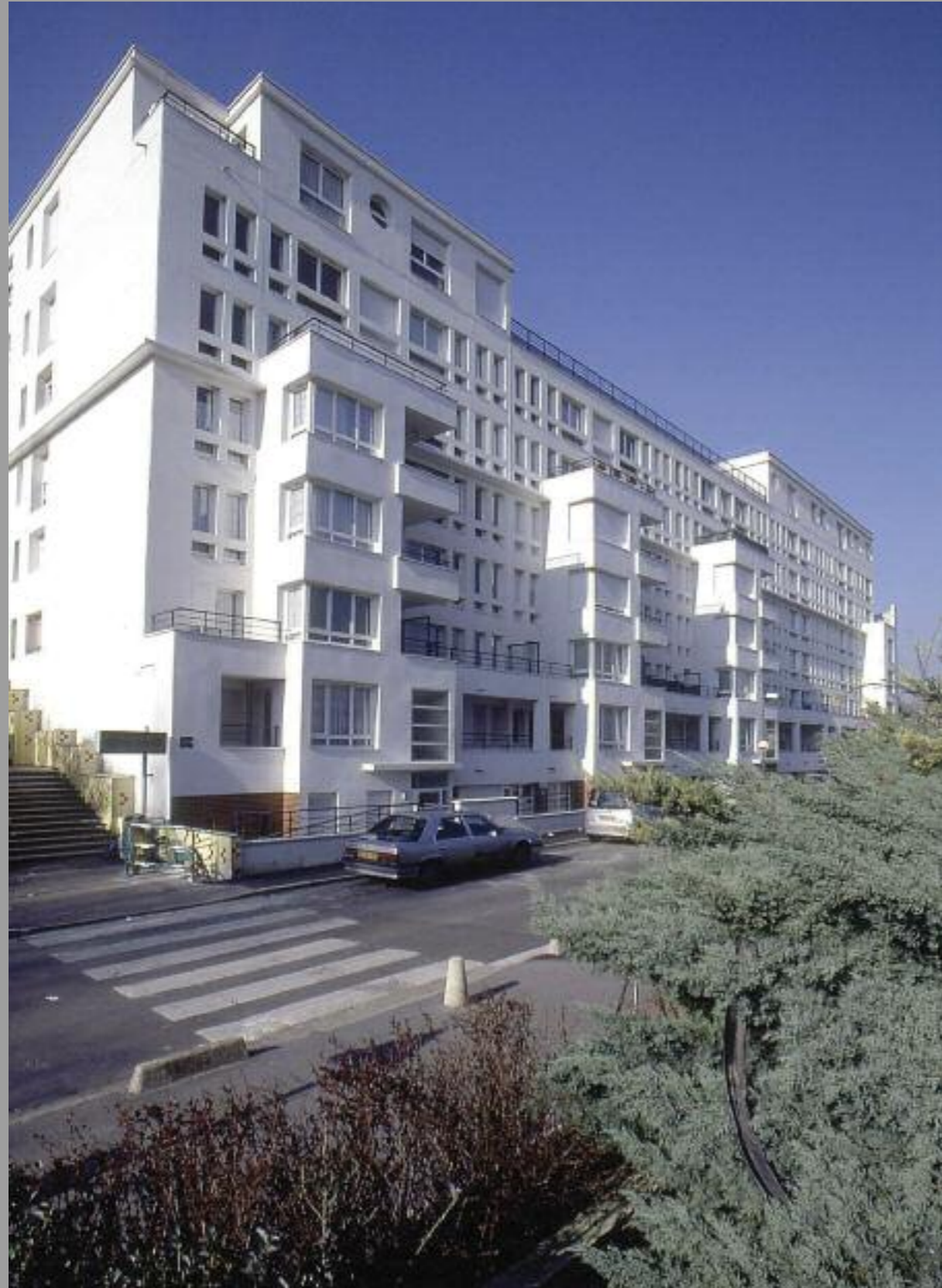
REMODELAGE BARRE DIDEROT VAL d'ARGENT, ARGENTEUIL, 2001
